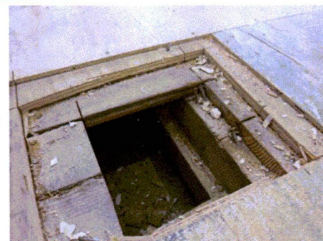
Figure 8 – Courtroom Floor Assembly
