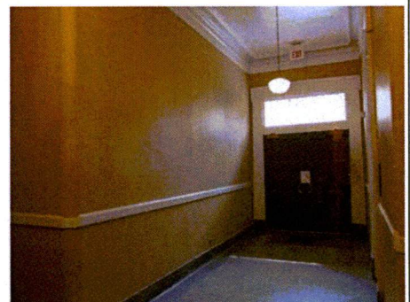
Figure 6 – Interior Plaster (East Wing)
