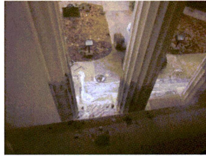
Figure 2 – Exterior Plaster (Columns)
